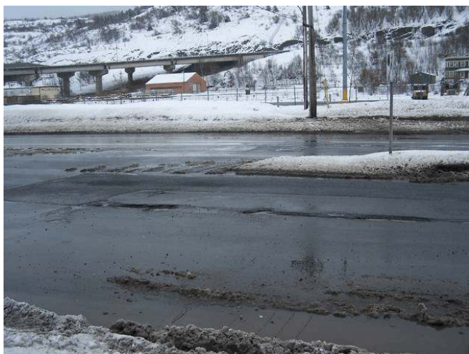
Photo taken by author of pothole showing streetcar tracks on Water Street in February 2008.
