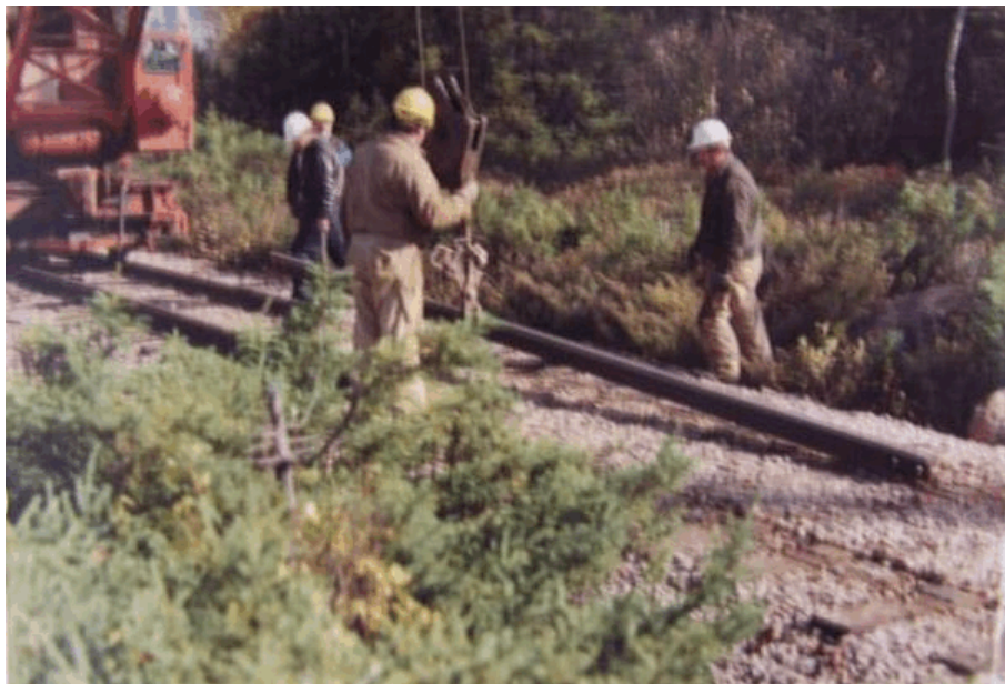
Work crew dismantling railway tracks in Newfoundland, Fall 1988.
